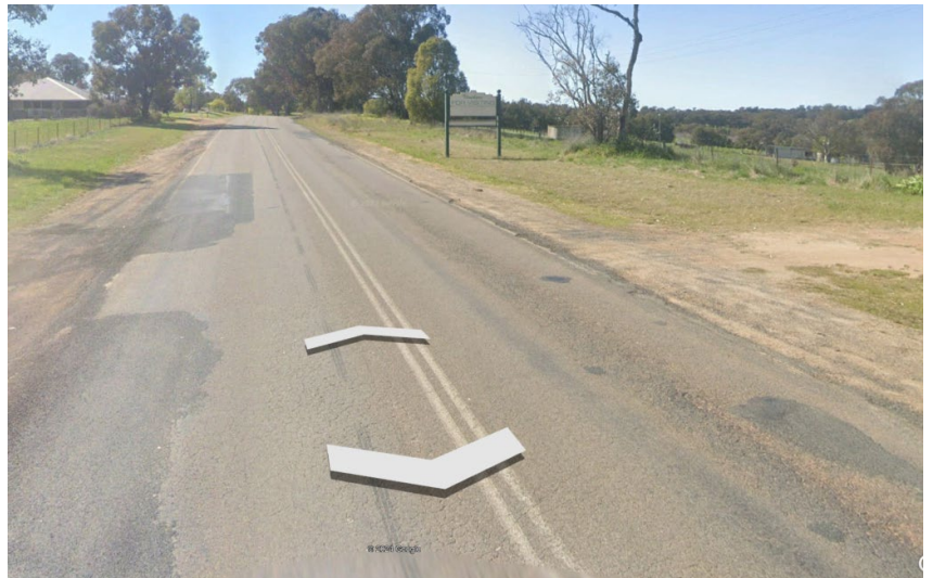
Figure 2.7: Murringo Road (Source Google Earth, December 2024)
